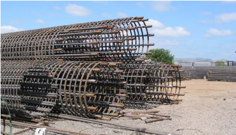
HRC 490 Position Couplers used to connect pre-tied reinforcement
