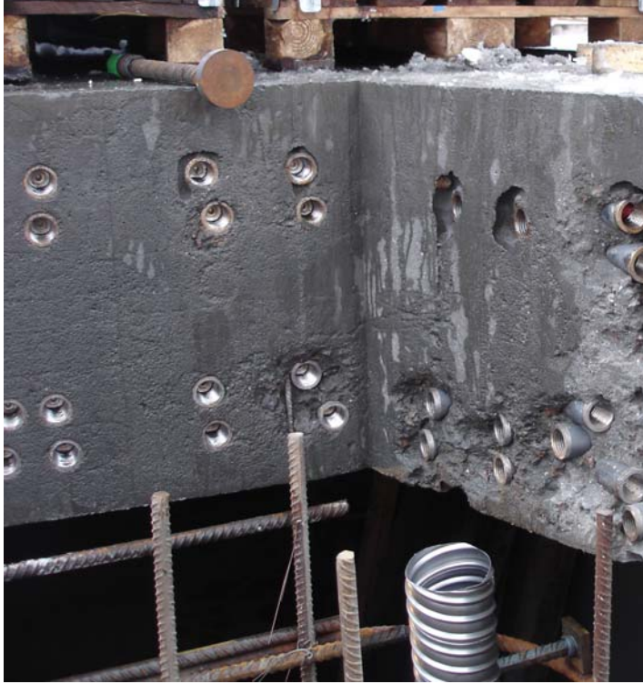
Improved accessibility by avoiding protruding rebar
