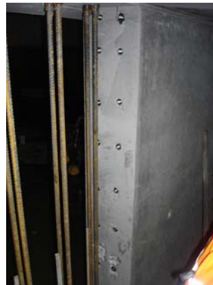
Subsequent closing of opening for prestressing equipment
