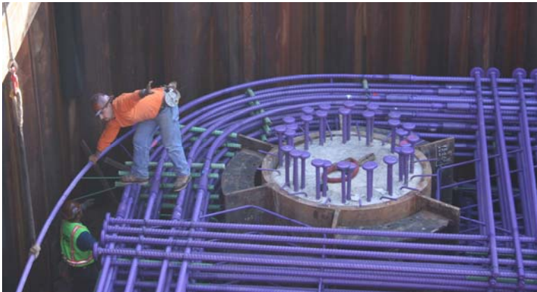
HRC 490 Position Couplers for bend rebar
