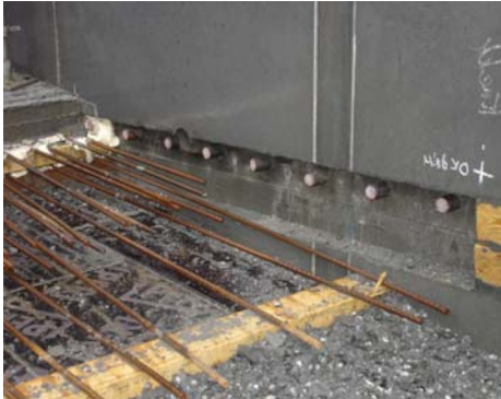
Detail of slab-wall connection
