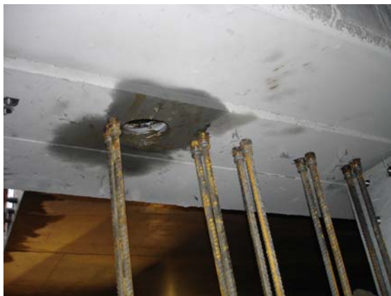
Subsequent closing of opening for prestressing equipment
